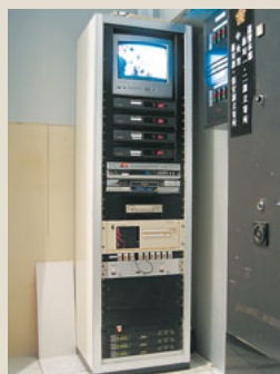
The video sources are installed in an equipment box beside the entrance.
